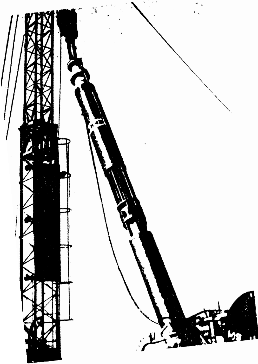
Fig. 6: submersible motor pump mode of installation
