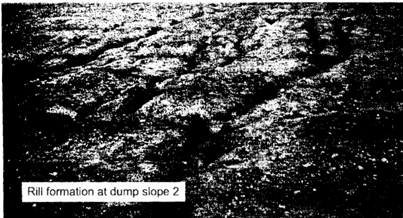
Figure 6: Water erosion patterns at lake embankment (dump slope 1 and dump slope 2) consisting of overburden materials.
