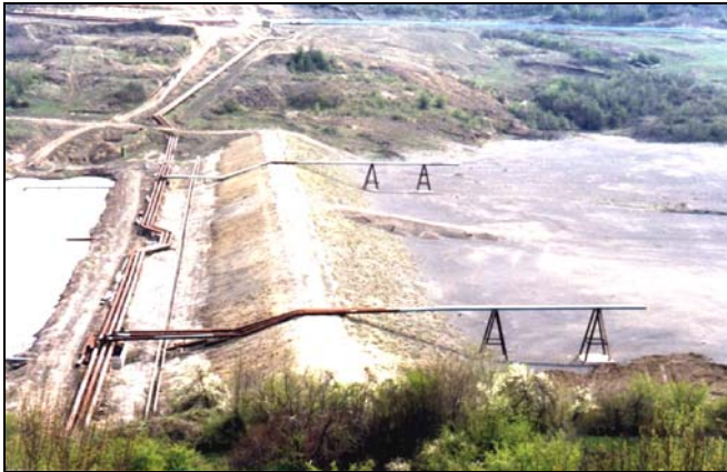
Photo 2 Way of placing the ash by hydraulic means
