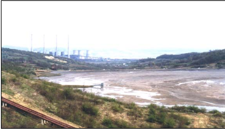
Photo 1 Total situation of the fly ash deposits
