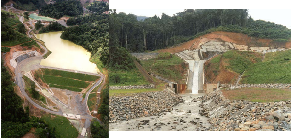
Photo 3: Santong #2 sediment control structure.
