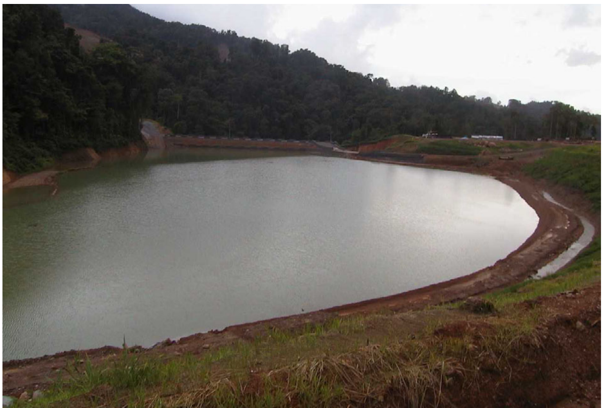
Photo 2: Santong #1 sediment control structure.
