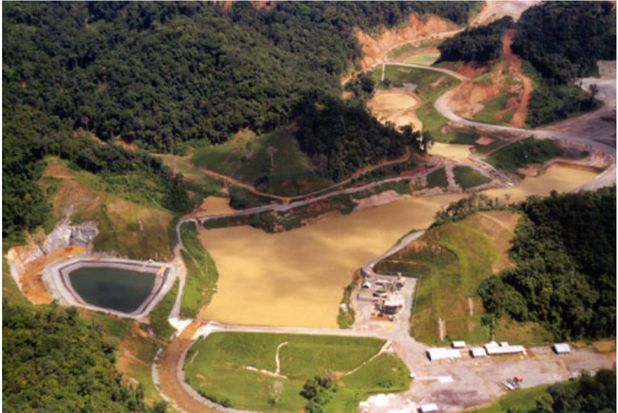
Photo 1: The Tongoloka toe dike, water treatment plant and pond.
