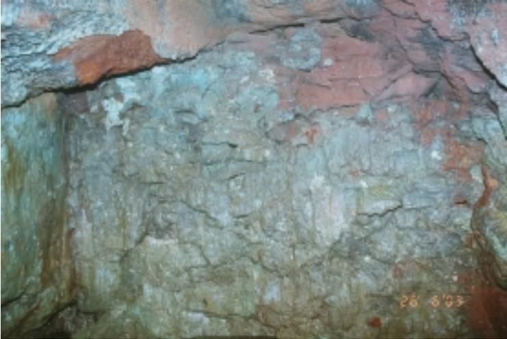
Figure 23: Stable face (gneiss plates in the vein region)
