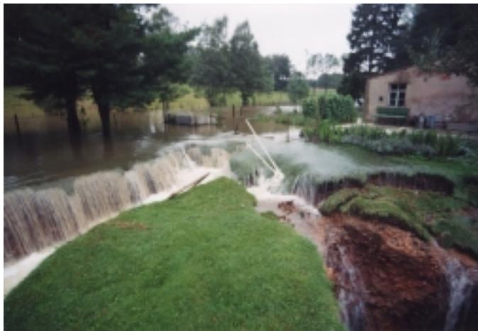
Figure 4: Breakthrough of the creek "Muenzbach" into old openings
