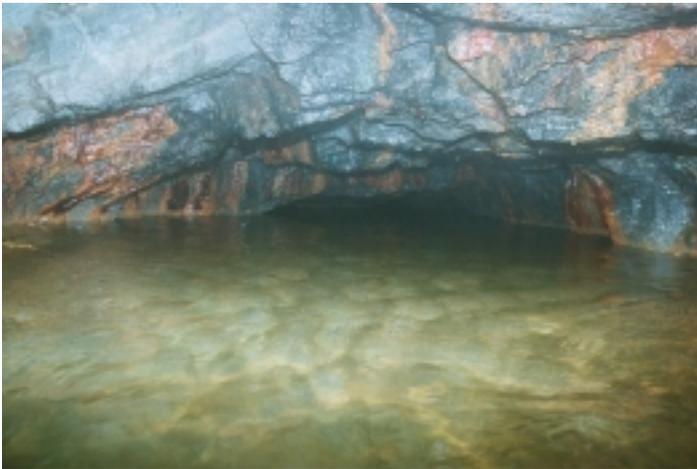
Figure 12: Rock mass and water filling the entire cross-section in the bypass
