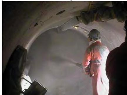
**Figure 8:** Example of shotcrete plug at Febex experiment [7]
