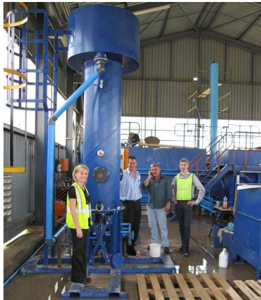
Picture 5. Crystalactor pilot plant at Gold Fields Driefontein’s mine
