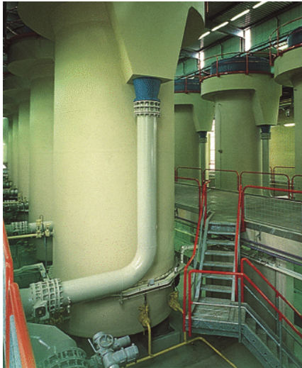
Picture 3. Crystalactor for softening of drinking water, Municipal Drinking Water Company of Amsterdam, The Netherlands. Capacity: 8,500 m 3 /h
