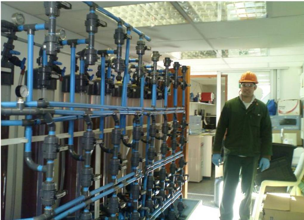
Figure 3. IX column and manifold arrangement for Earth pilot plant
