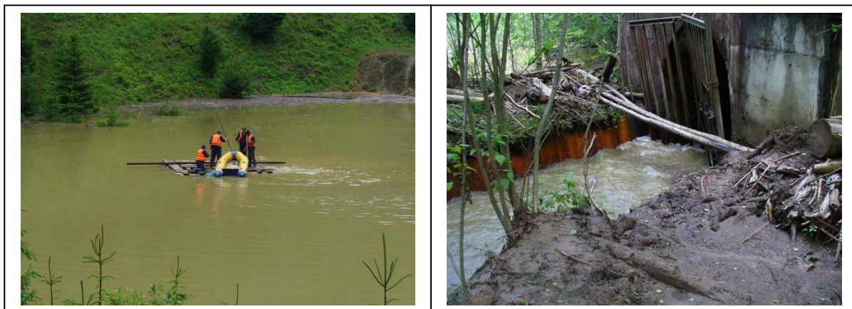
Figure 4. Temporary lake formed on the top of the tailing dam endangering the downstream inhabitants and tourists located in Ostra village (detail of the diverting tunnel of the creek from the upstream area of the tailing dam, partially blocked with debris)
