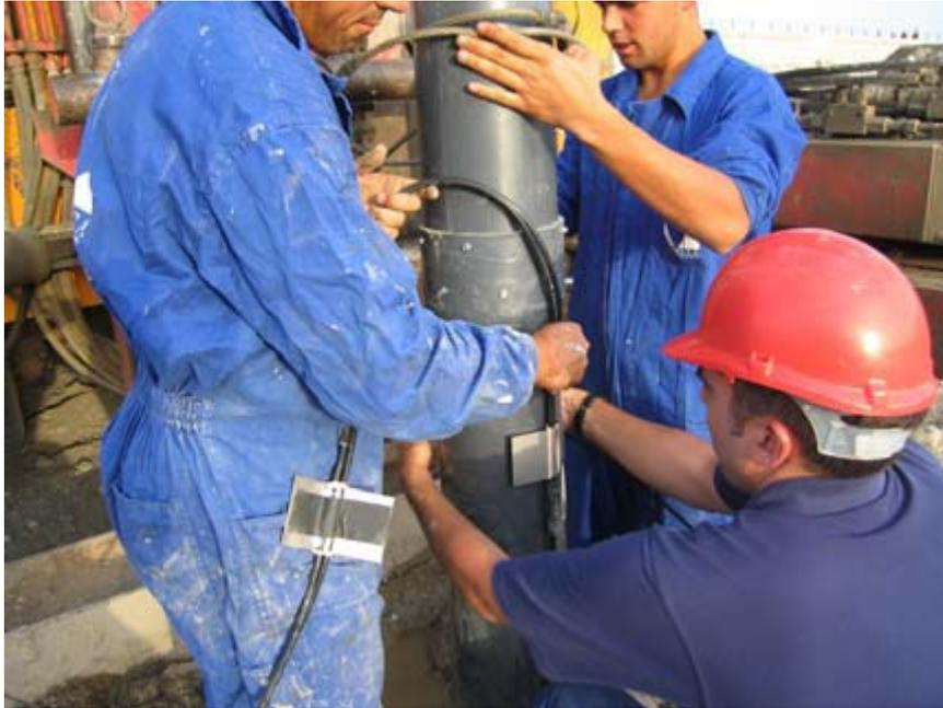
Fig 3. Attaching downhole electrodes to borehole
