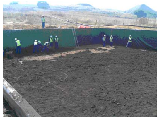
Plate 2. Filling of DPBR with Carbon
