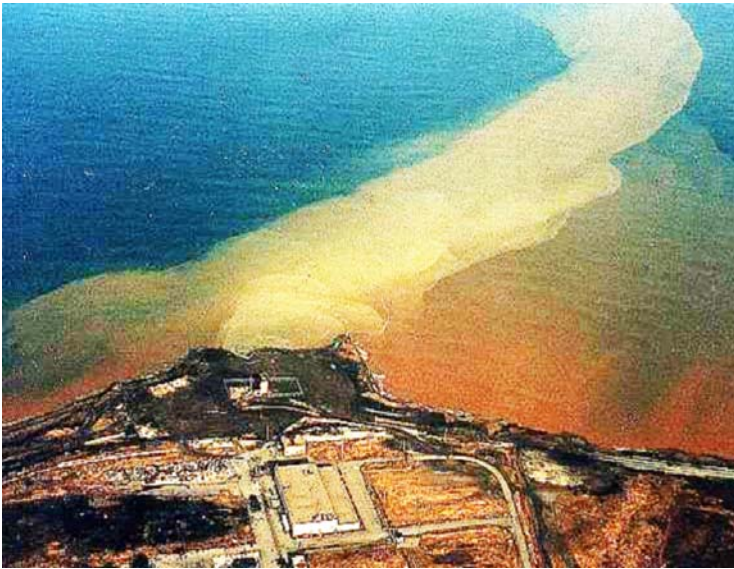
Figure 5 – Iron rich plume from the 1B System at the 1B Shaft
