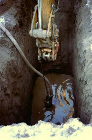
Figure 3 Investigation of the subsoil by trenching Figure 4 Sampling of the groundwater to the perpetuation of evidence
