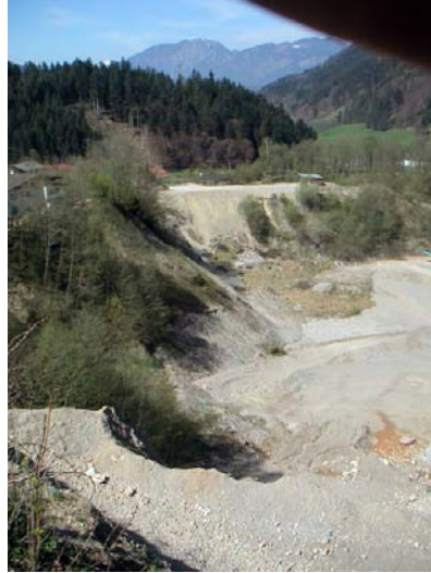
Figure 2 Scrap view of the open-pit mine before refilling
