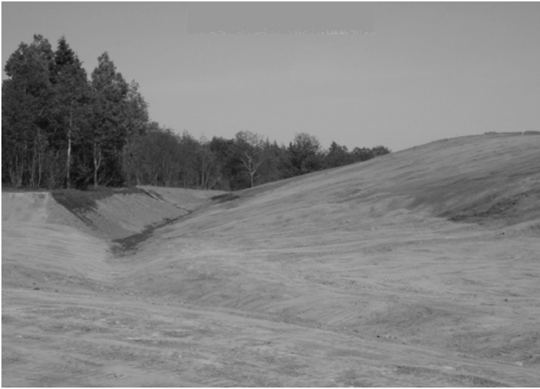
Figure 2 View of the re-profiled pile prior to placement of the engineered cap
