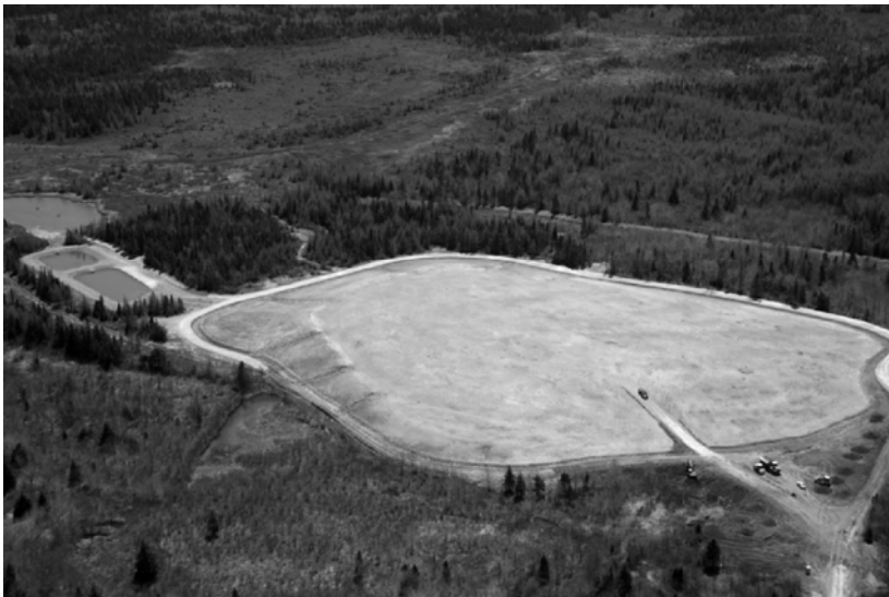
Figure 3 Aerial view of the reclaimed waste rock pile, May 2010
