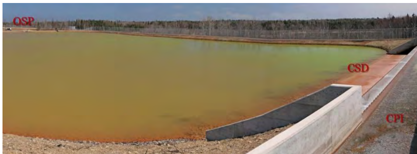
Figure 1 Sampling locations CPI (Cascade Pond Inflow), CSD (Cascade Settling Pond Discharge), and OSP (Outflow Settling Pond) in the order of the flow direction at the Neville Street Wellfield. Flow through the settling pond is from right to left. Image taken in 2006.
