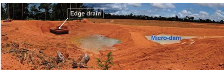
**Fig. 6** Micro-dam built on drainage channel.
