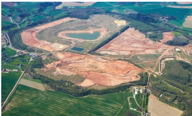
Fig. 1 Aerial photograph of the Culmitzsch TSF with pond A (left, with supernatant water) and pond B (right) and the Lokhalde waste rock dump (centre foreground) during remediation (2012).
