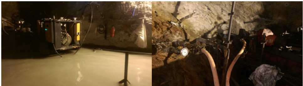
Figures 2 & 3. Left: Test terminated early as water levels reached the pre-arranged shut-in trigger level. Right: Example drain holes with manual read pressure gauges and 2 open holes with hoses attached for barrel-fill flow rate tests.
