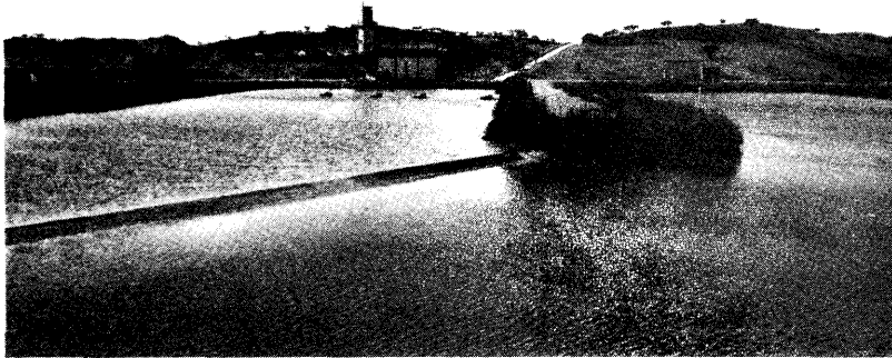
SURFACE TREATMENT PLANT (Lagoons 1 and 2)
