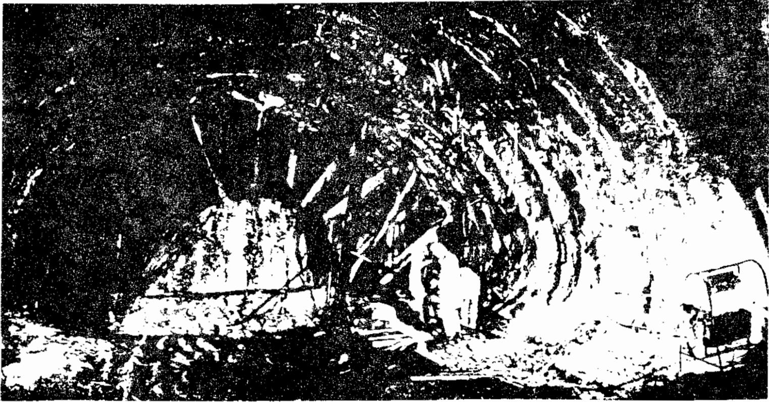
Fig.2: Temporary support measures in the tunnel at the location of the first water inrush, station 732 m
