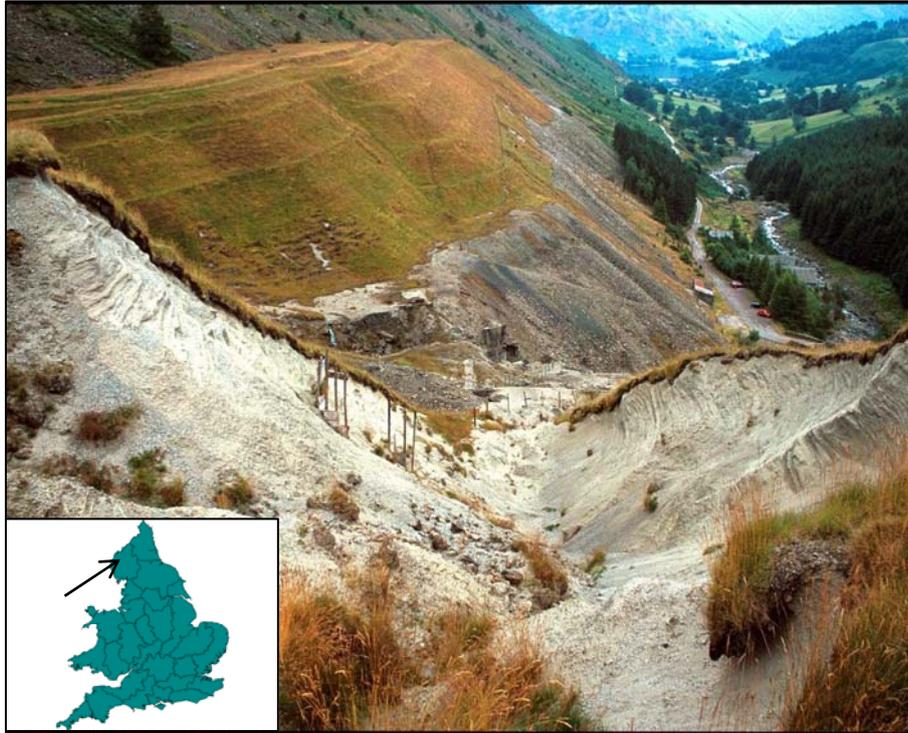
**Fig. 1.** Location map for Greenside Mine, and view east towards Ullswater showing collapsed tailings dam and erosion of spoil heaps
