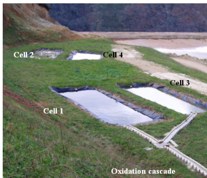
Fig. 1. View of the in-situ pilot-scale system.
