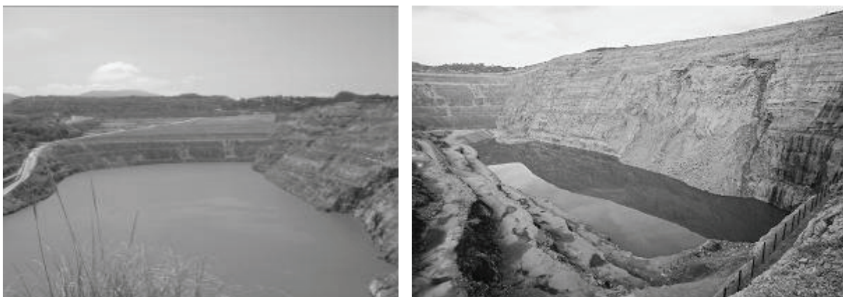
Figure 5. Two different phases in the open pit filling (Right, elevation 0 meters; Left, elevation +13 meters above sea level).
