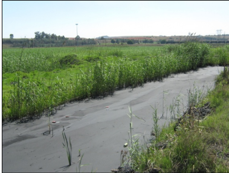
Figure 2. Silting up of dirty water canal
