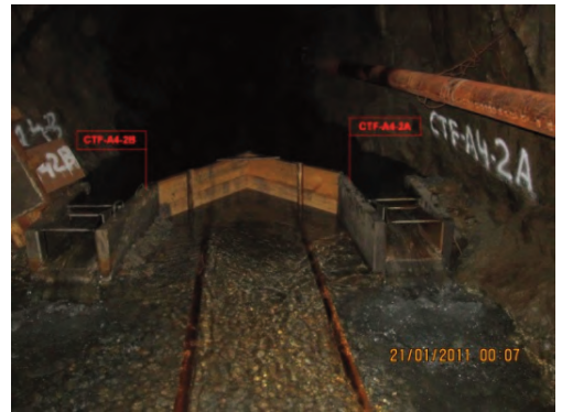
Figure 8 Second concrete flume box and more expansive levee stations CTF-A4-2A and 2B.
