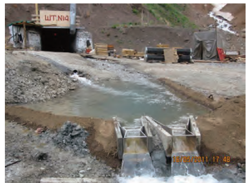
Figure 9 Discharge from Adit 4.
