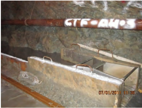
Figure 5 Baski flume in concrete flume box; note the tight fit between the rib of the drift and cart track.
