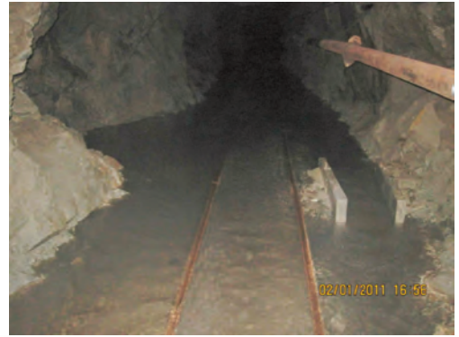
Figure 7 Increased flow following borehole testing overran capacity on the Baski flume at CTF-A4-2.
