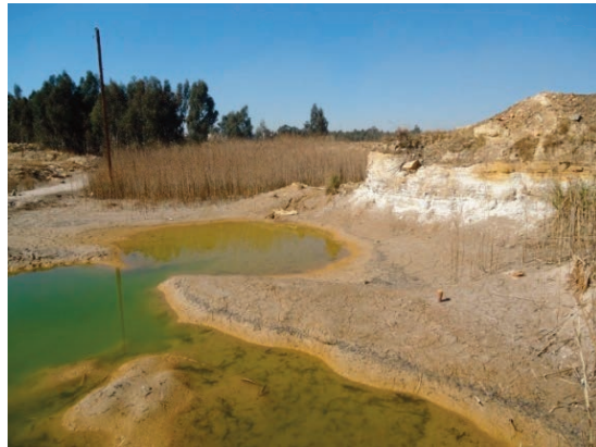
Fig. 1 The edge of an abandoned tailings storage facility with efflorescent crust on the wall
