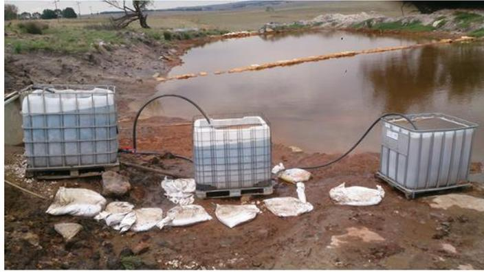
*Figure 2 Carolina pilot passive treatment RAPS and oxidation units*
