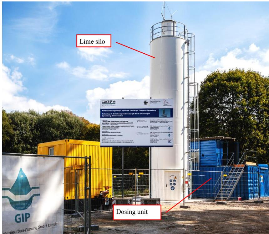
**Figure 2** Container-based mobile plant providing tailored lime slurry dosing (Plant Unit 1)
