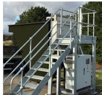
**Fig. 4** Soneco® Sono-electrochemical water treatment for removal of Phosphorus from wastewater
