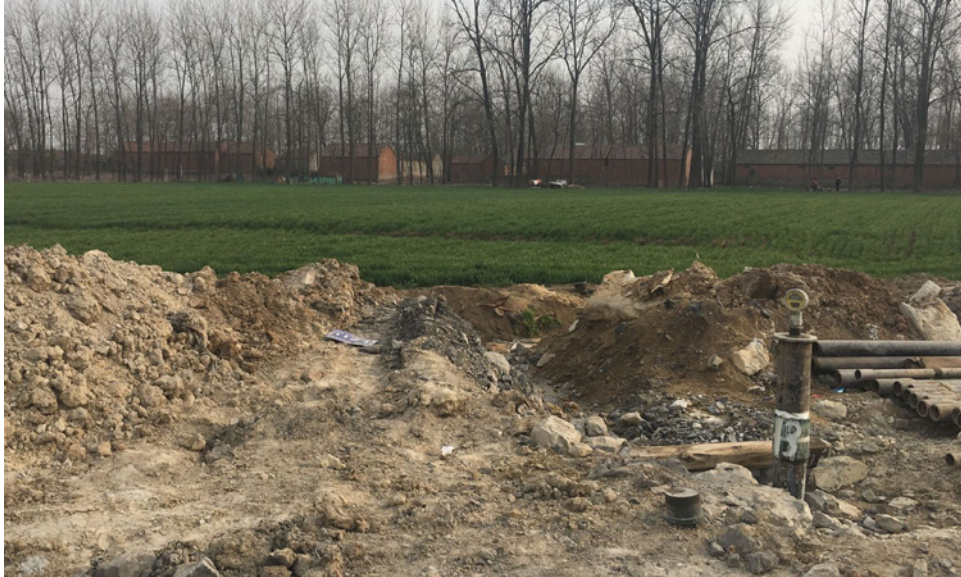
Figure 5 The surface around the grouting drilled
