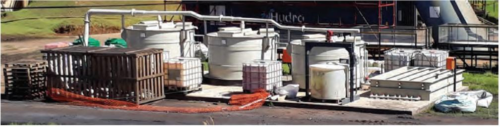
Figure 1 A view of the installed biological sulphate reduction pilot plant
