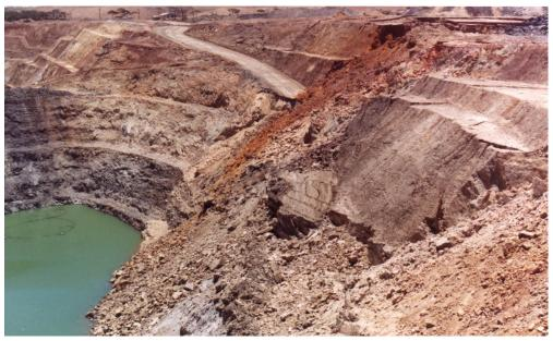
Photograph 2: Structural failure in weathered to fresh Archaean rock
