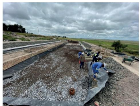
Figure 3 Refurbishment of the first pond (RAPS 1) (left) and compost mixed with limestone in RAPS 1 (right).
