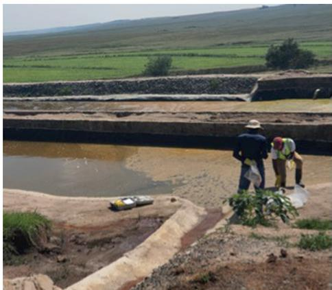
Figure 4 An overview of RAPS 1 showing channeled inlet water, ponded mine water under treatment and a berm in the center (for increasing retention time).
