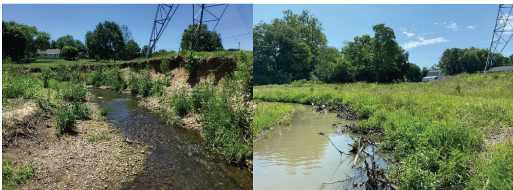
Figure 5 Bank Height Comparison for Unstable (Left) and Restored Stream (Right)
