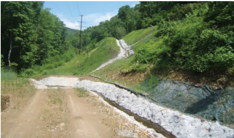
Figure 1 Riprap used for Conveyance on Reclaimed Land in West Virginia
