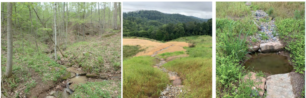
Figure 2 Reference Reach (Left) and Constructed Step Pools (Right) for Headwater Streams
