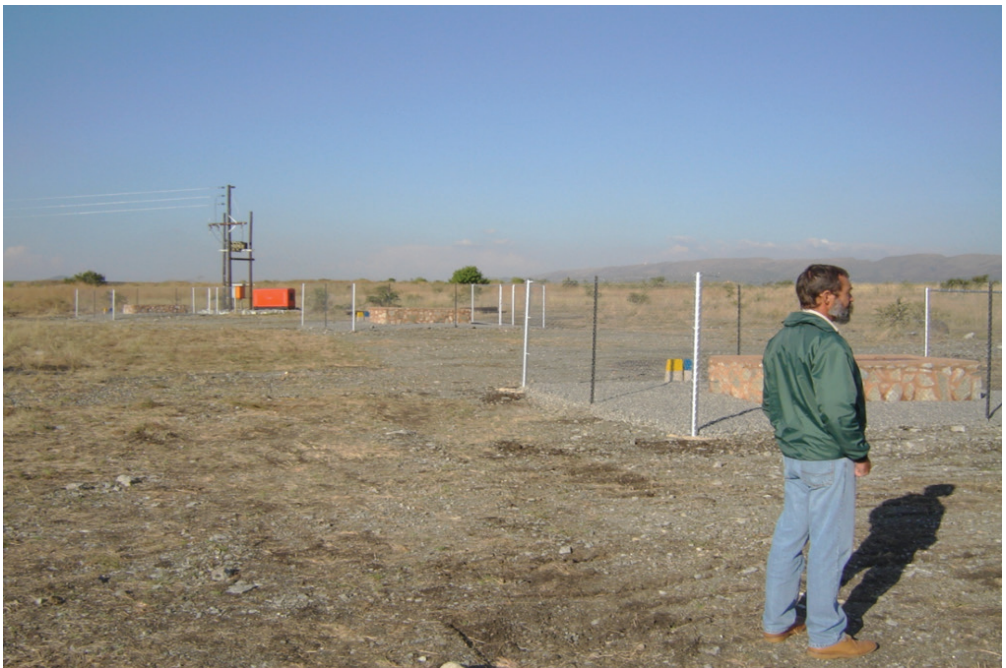
Figure 1 A photo of a rehabilitated open pit mine near Rustenburg, South Africa. It is filled with backfill material covered with topsoil. It also shows three boreholes drilled into the backfill material pumping freshwater from the pit to be re-used rather than taking water from nearby agricultural irrigation channel (image: Botha et al 2011).
