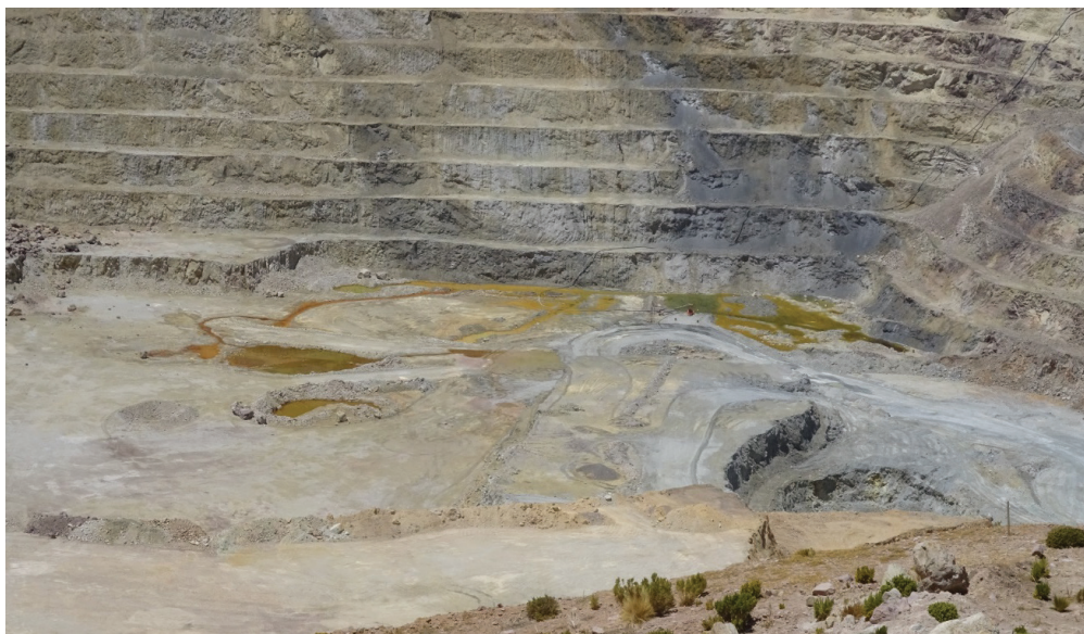
Figure 1 Pit floor flooding due to seepage.
